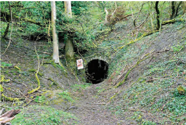
The short surviving limestone adit.
